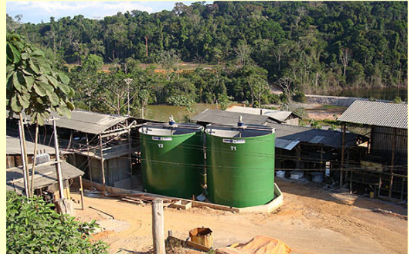
Leach tanks for CIP expansion are complete and being commissioned
